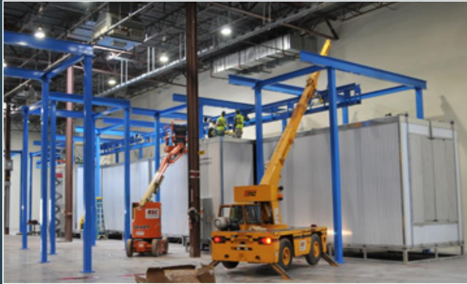
*Modular construction allows for installation in half the time of conventional systems*
